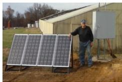
About four years ago however, we replaced the problematic AC power distribution system with a solar panel power system and added extensive grounding to the tower in the process. After that was done, the Crofton microwave link stayed up for over three years before lightning once again destroyed the radios. Damage to equipment at ground level was negligible however.
